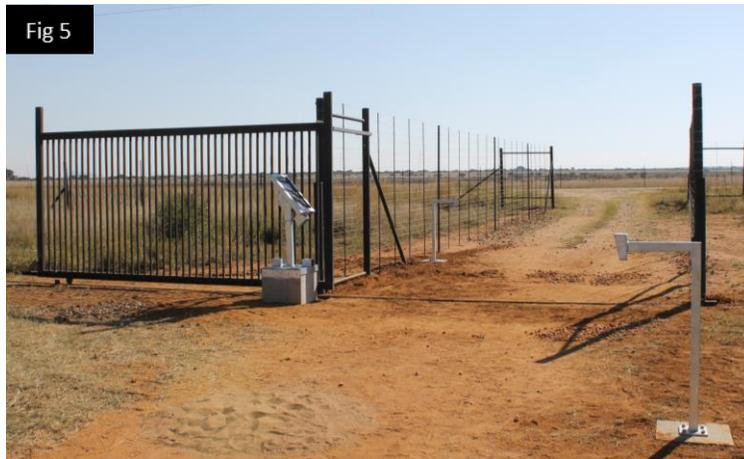
**Fig 5** shows the sliding gate in its fully open position. Two goosenecks have been installed, each fitted with keypads to open the gate.
