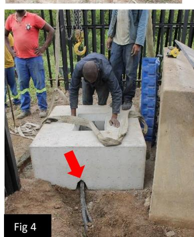
**Fig 1** shows a newly installed Borehole Vault, consisting of an outer shell and a central lid, made from 60MPa concrete, and weighing 1.4 tons. These vaults are replacing steel 'box & lid' chambers that are currently being vandalised, see **fig 2**.
